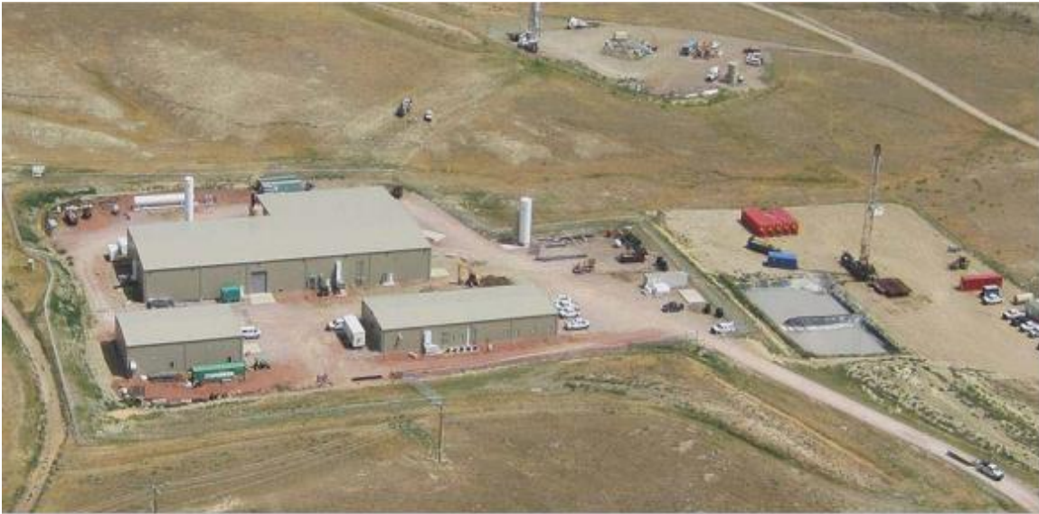
Nichols Ranch Processing Facility, Powder River Basin, Wyoming
